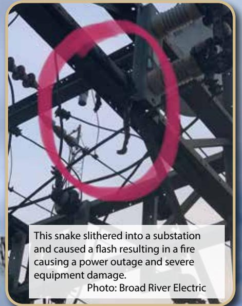
This snake slithered into a substation and caused a flash resulting in a fire causing a power outage and severe equipment damage.
